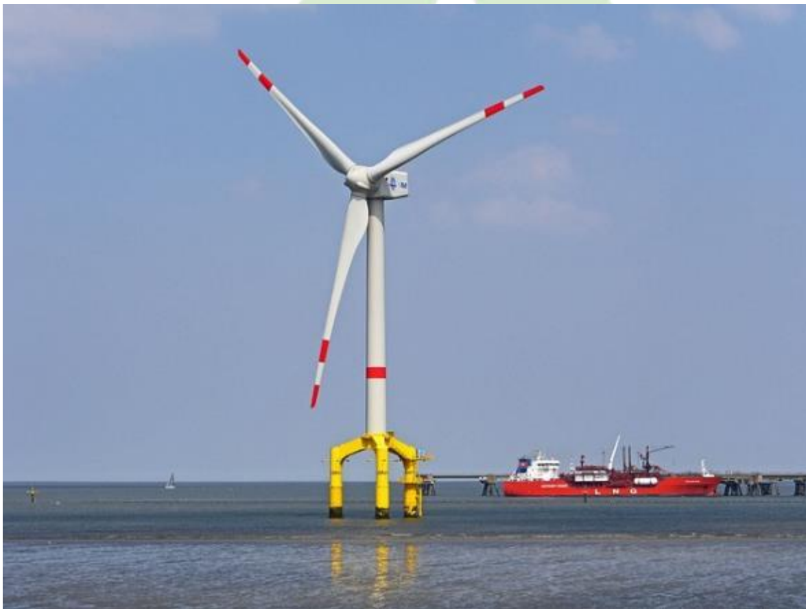
TURBINA EOLICA OFFSHORE
